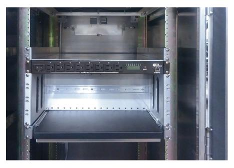
The ITS Commander is designed to improve system reliability and lower the cost of ownership through reduced maintenance costs. The system benefits both the owning agency and maintaining agency by promptly sending signals of an abnormal situation, allowing routine monitoring of critical equipment, and providing the capability to remotely control outlets to reboot equipment, if needed. These features can reduce unnecessary trips to inspect or service the cabinet and saves money.
